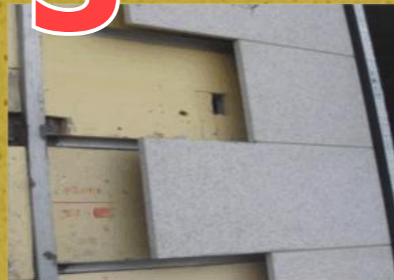
Traditional Stone Curtain Wall System
